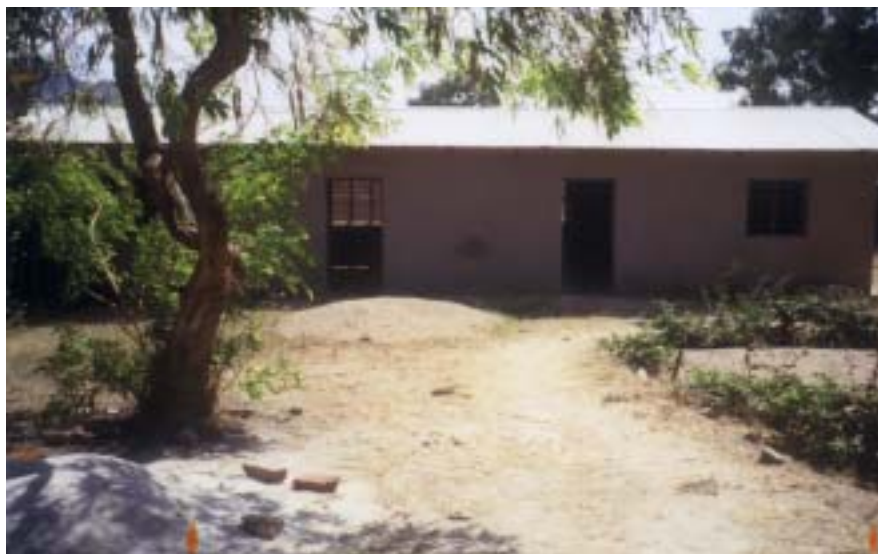
The laboratory building, recently completed, at the Ilula Health Centre
