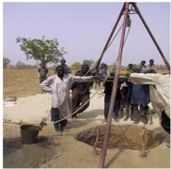
A well under construction, partially funded by GHM.
