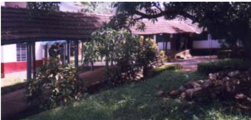
Major renovation of Karunalya Hospital in Kerala, India was made possible through a matching grant program with LCMS.
