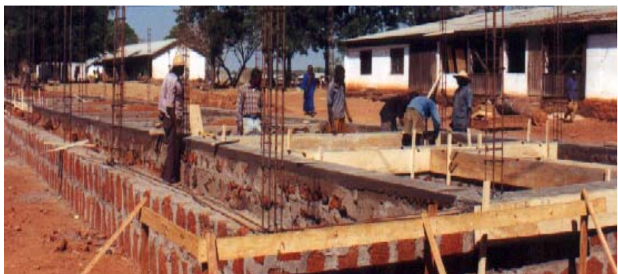
Construction of additions to hospital facilities took place in several countries.
